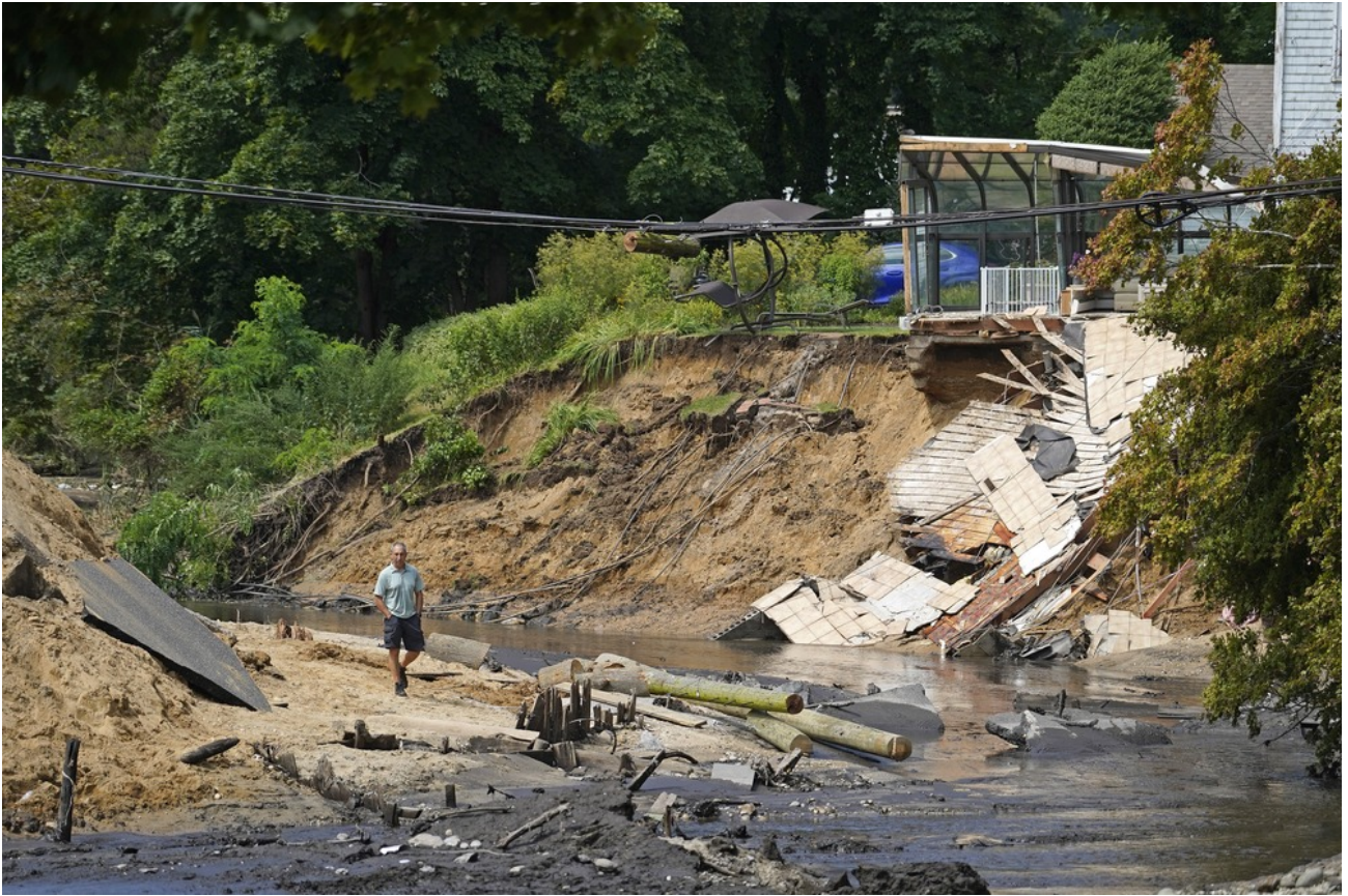
A man walks on the dirt and sand foundation of Harbor Road in Stony Brook, N.Y., Aug. 19, 2024, after it collapsed earlier in the day when torrential rain caused a dam beneath the road to burst. The storm unleashed flash floods in parts of Long Island, N.Y., and southwestern Connecticut, where two women were found dead after they were swept away from their vehicles. (OSV News/Gregory A. Shemitz)
