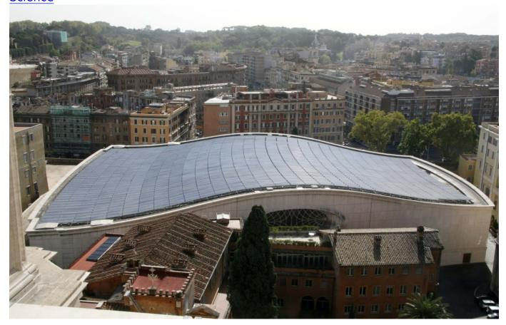
Solar panels cover the roof of the Vatican's Paul VI audience hall in this photo released by the Vatican in 2008. The hall's original concrete roof was replaced with panels of photo-electric cells, generating the city's first solar power. (CNS/Vatican)
