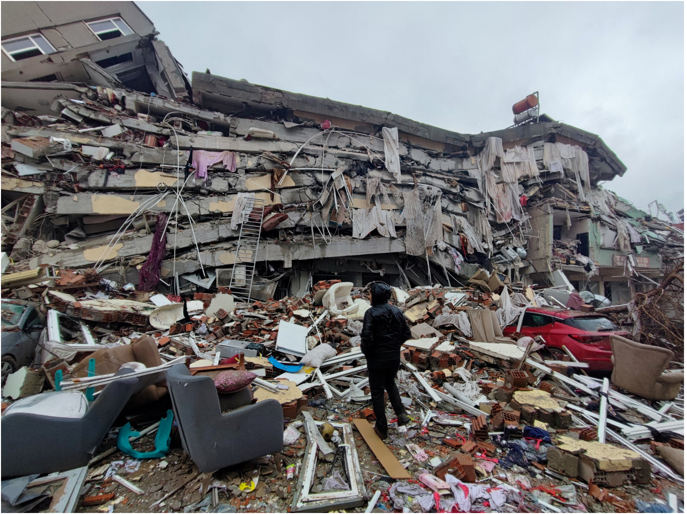
A man stands in front of collapsed buildings following an earthquake in Kahramanmaraş, Turkey Feb. 6, 2023. A powerful 7.8 magnitude earthquake rocked areas of Turkey and Syria early that morning, toppling hundreds of buildings and killing more than 2,000 people. (OSV News photo/Ihlas News Agency via Reuters)
