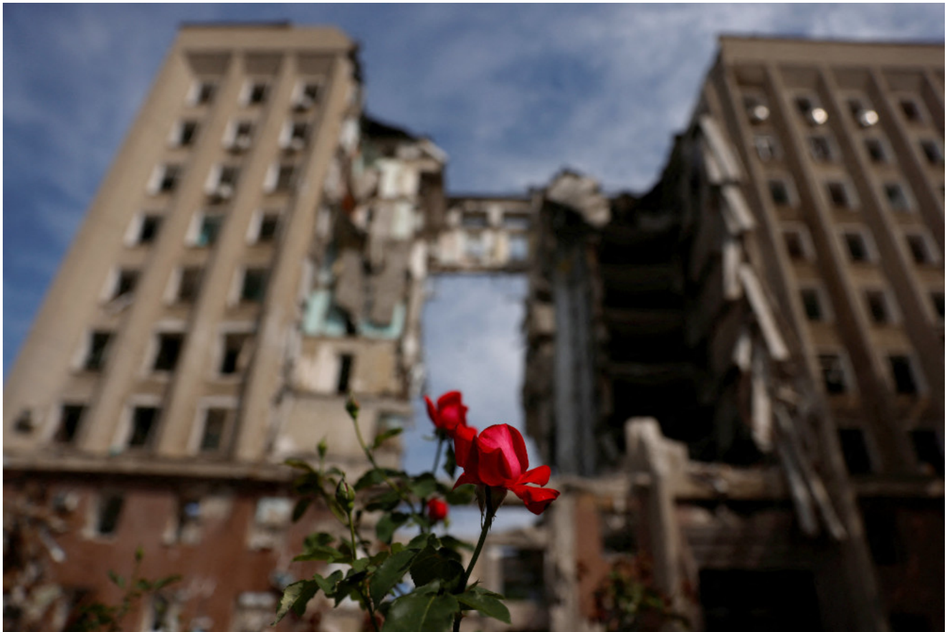
A flower is pictured in front of the destroyed regional administration building following shelling by Russian troops in Mykolaiv, Ukraine, June 8. (CNS/Reuters/Edgar Su)
