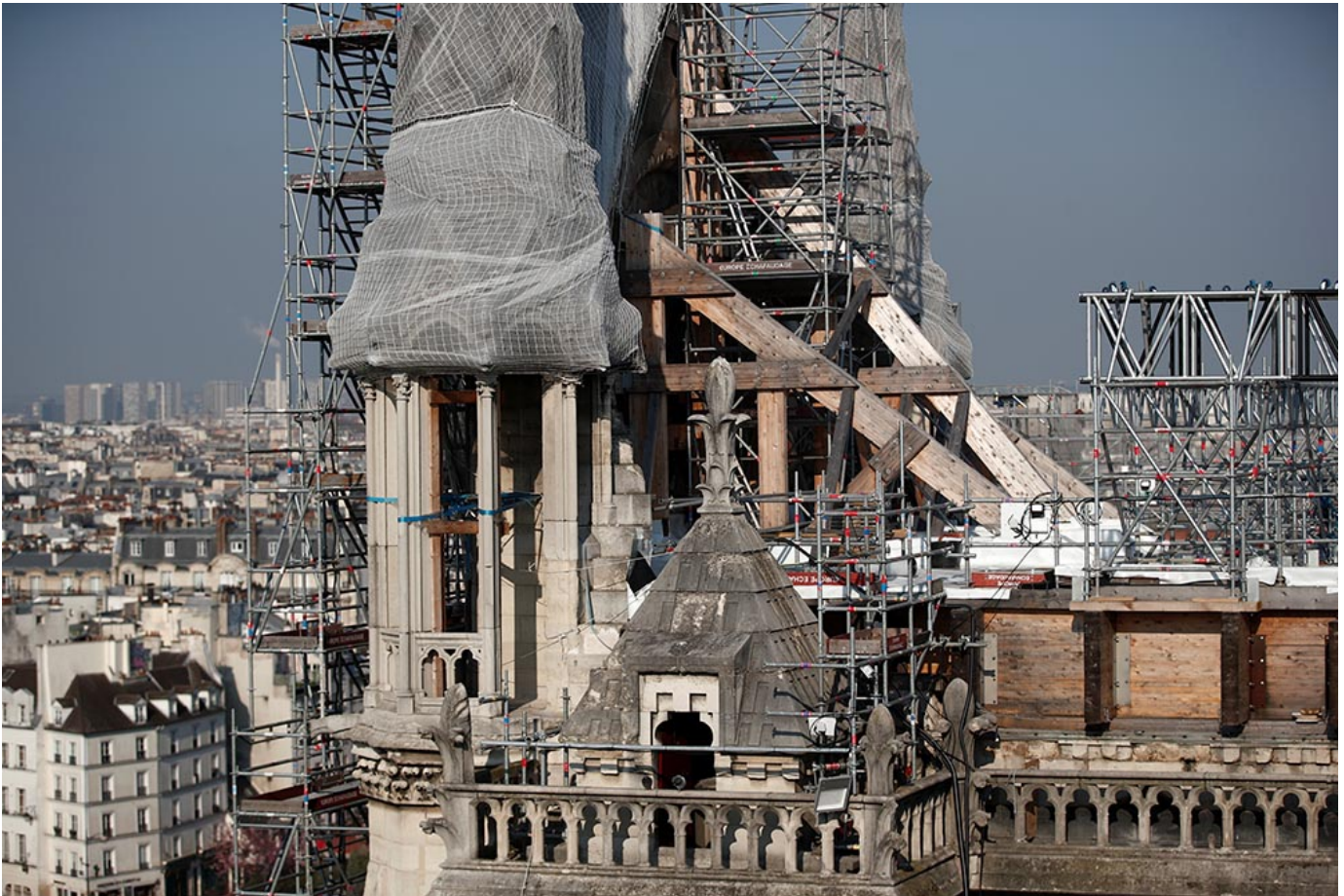
Scaffolding surrounds the damaged Notre Dame Cathedral April 15 in Paris. (CNS/Reuters/Benoit Tessier)
