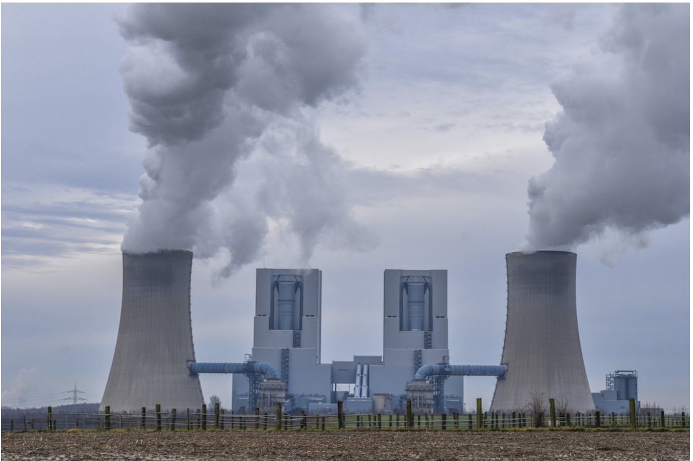
Coal-fueled power plant (Pixabay/Michael Gaida)
