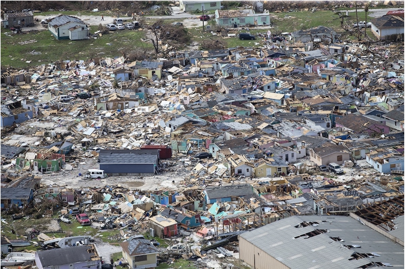
Destruction from Hurricane Dorian is seen at Marsh Harbour in Great Abaco Island, Bahamas, Sept. 4, 2019. (CNS/Reuters/Miami Herald/Al Diaz)
