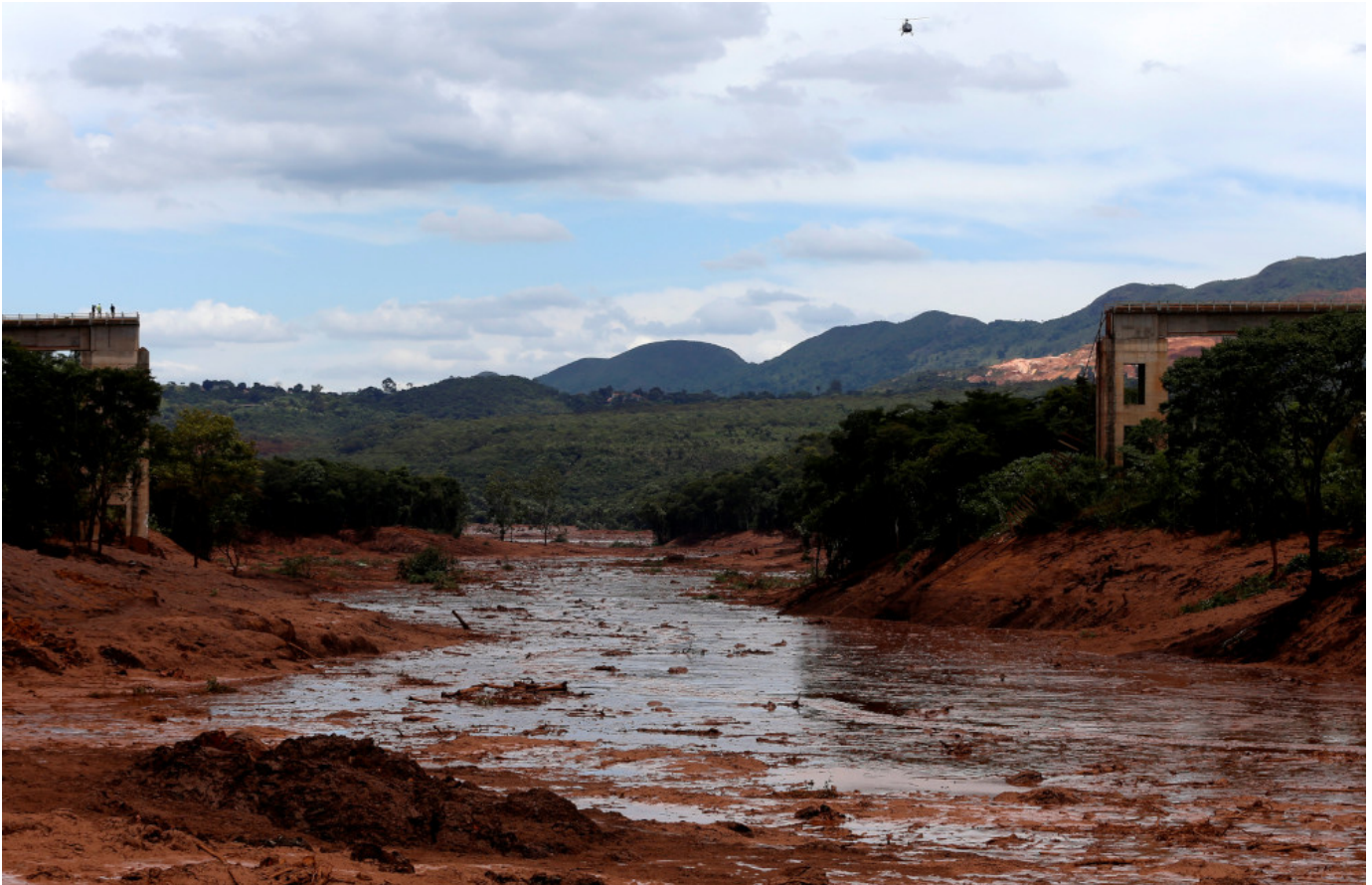
A view of the aftermath from a failed iron ore tailings dam in Brumadinho, Brazil Jan. 27, 2019. (CNS/ Reuters/ Adriano Machado)
