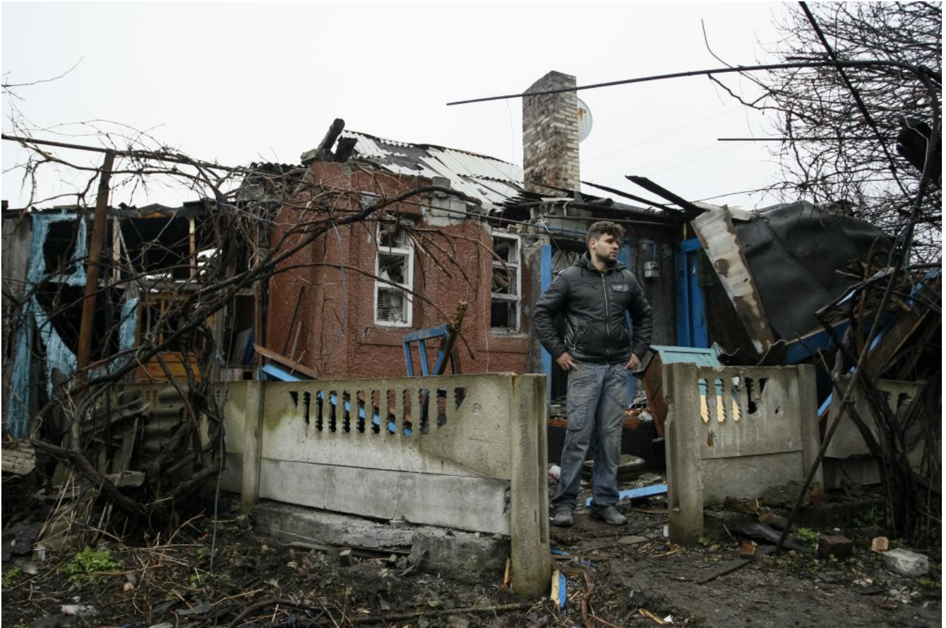
A man stands in front his damaged house after shelling March 24, 2016, in the Ukrainian town of Makeevka. (CNS/EPA/Alexander Ermochenko)
