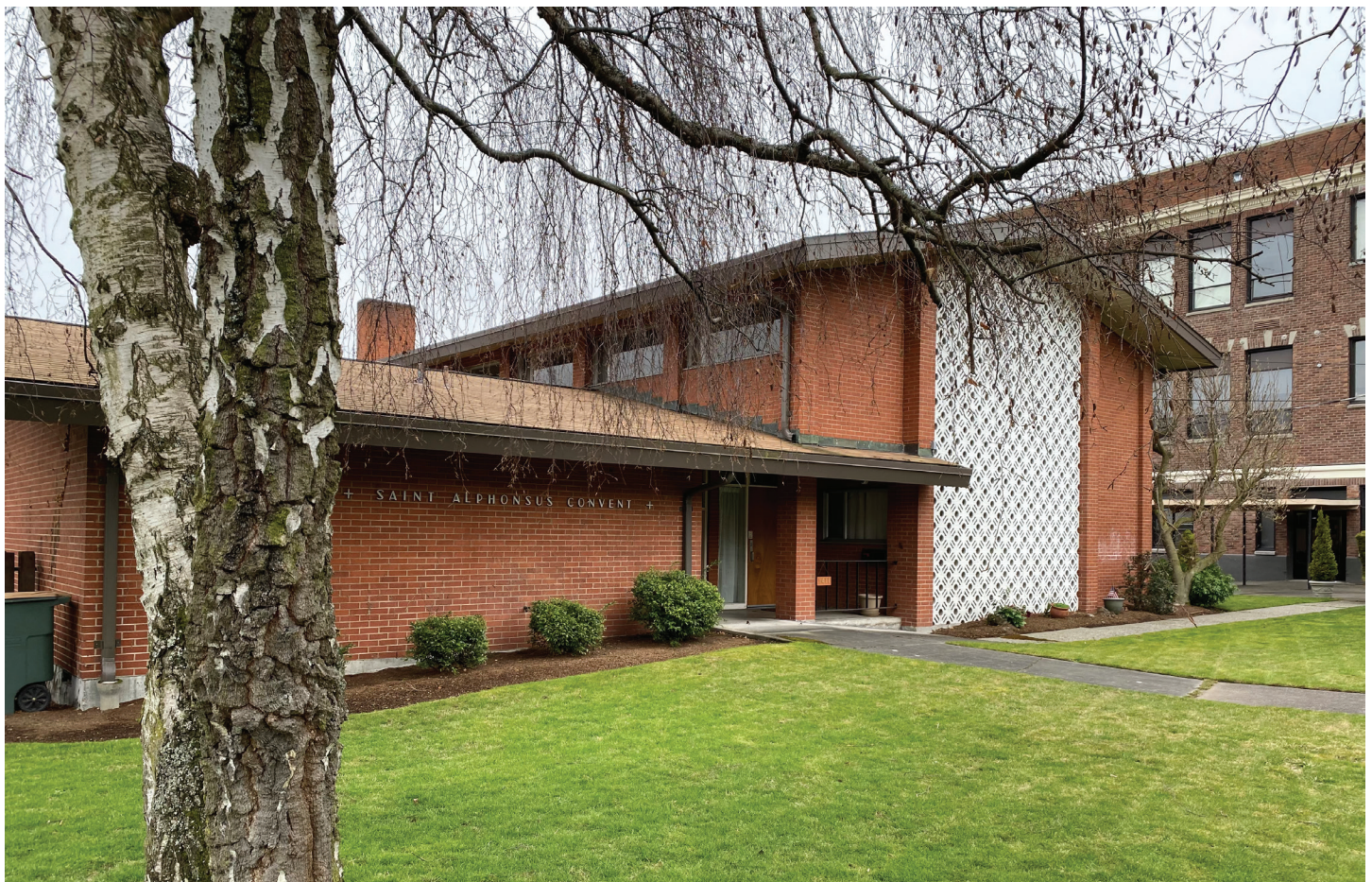
At St. Alphonsus Parish in Seattle, a convent once home to the Society of Our Lady of the Most Holy Trinity Sisters now houses Catholic school educators. Several U.S. dioceses are considering ways to repurpose their real estate into affordable housing for Catholic school teachers. (Courtesy of the Seattle Archdiocese)
