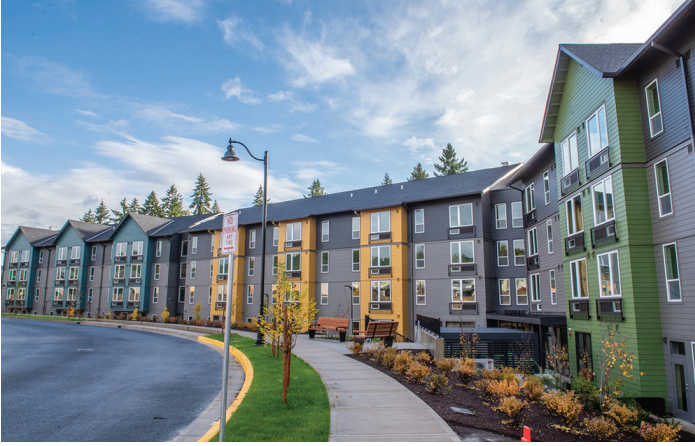
Good Shepherd Village, which opened Nov. 6 in the suburbs of Portland, has 142 units of affordable housing, including 58 units reserved for permanent supportive housing. With funding from a $652.8 million housing bond passed by Portland area voters in 2018, Catholic Charities of Oregon staff will provide supported residents with a range of services and case management. (Courtesy of Catholic Charities of Oregon)
