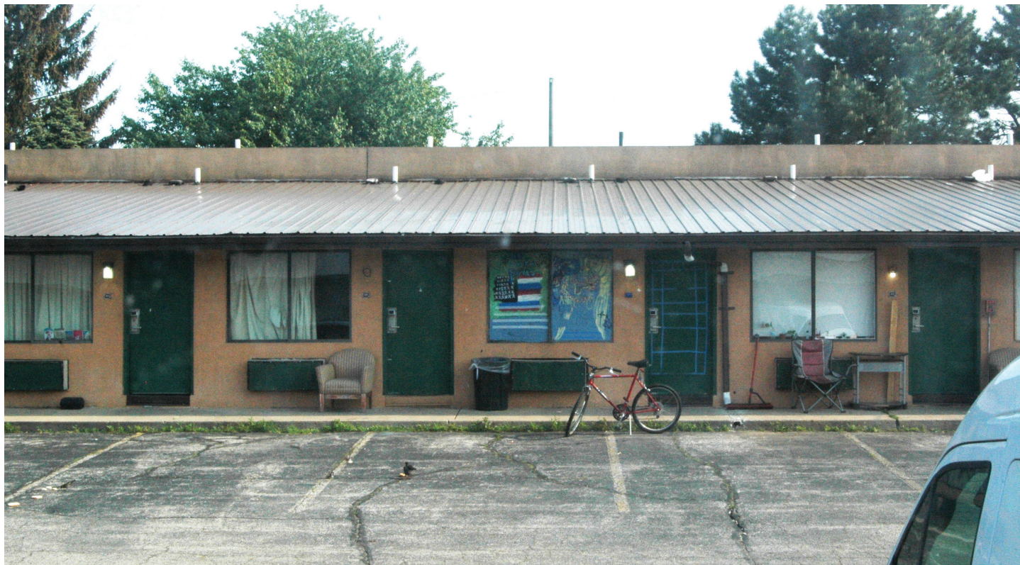
The outside of the renovated Knights Inn in South Bend, Indiana, that now houses the Motels4Now project to offer immediate housing to persons experiencing homelessness (Bill Odell)
